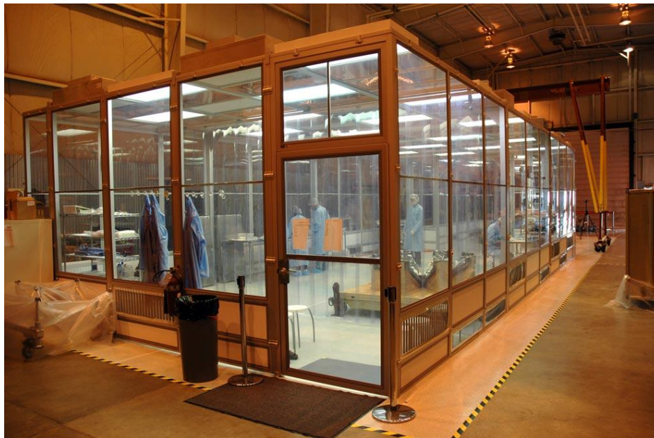
Figure 5-5: Genesis Temporary Cleanroom at UTTR (Image credit: NASA)
